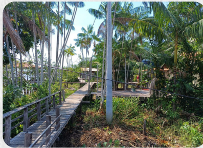
Example of pedestrian walkway: Jorocazinho community from above (photo: 11/14/2023)
